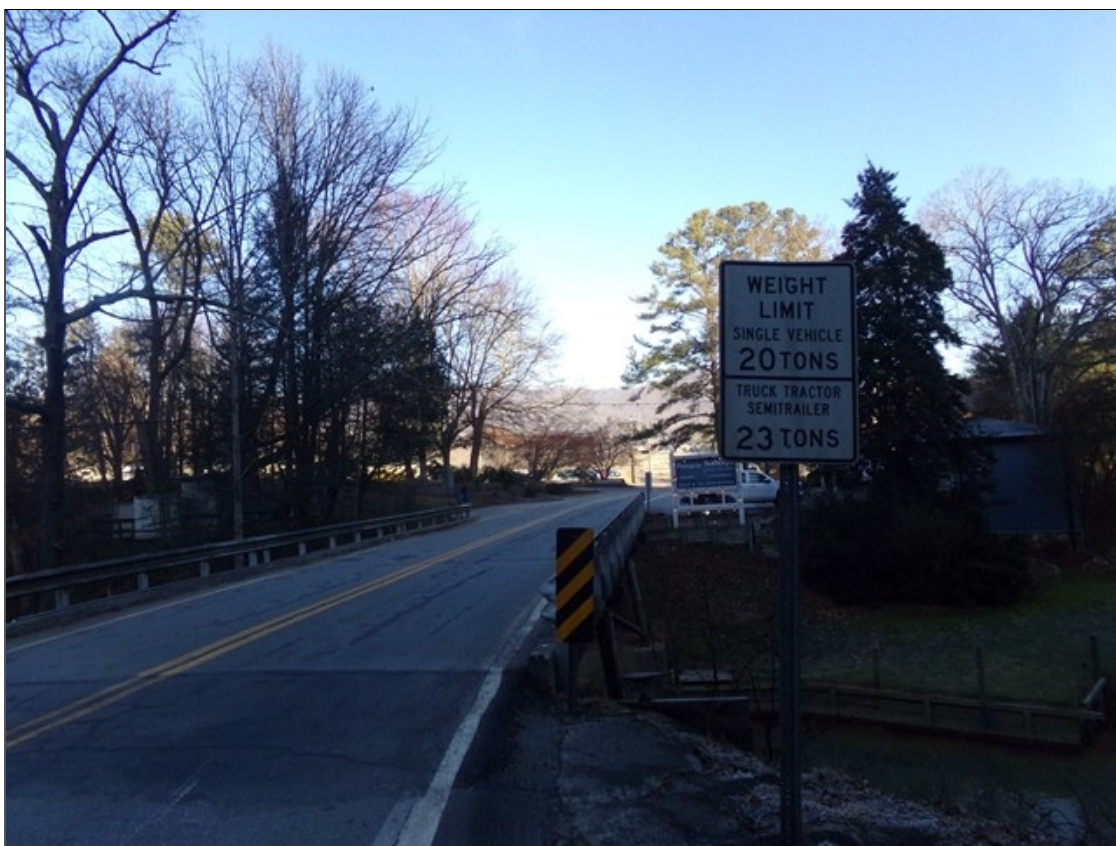
WEIGHT LIMIT POSTING AT SOUTH APPROACH
