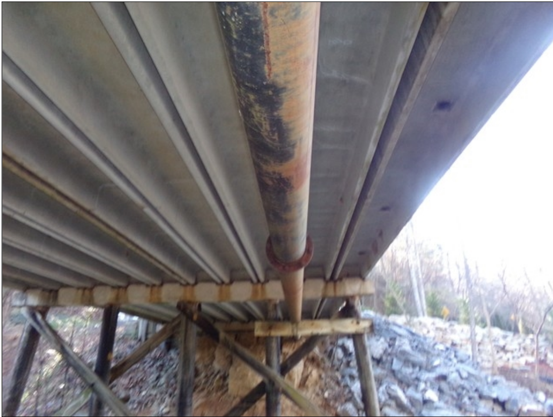
TYPICAL 10 INCH DIAMETER UTILITY BELOW BEAMS 2 AND 3 ALONG LENGTH OF BRIDGE (RESTS ON SUPPORTS AT BENTS)
