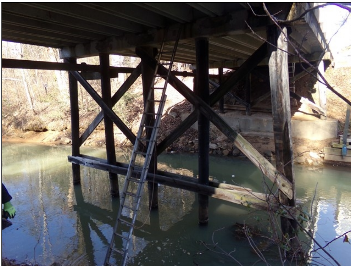
BENT 1, NEAR SIDE
