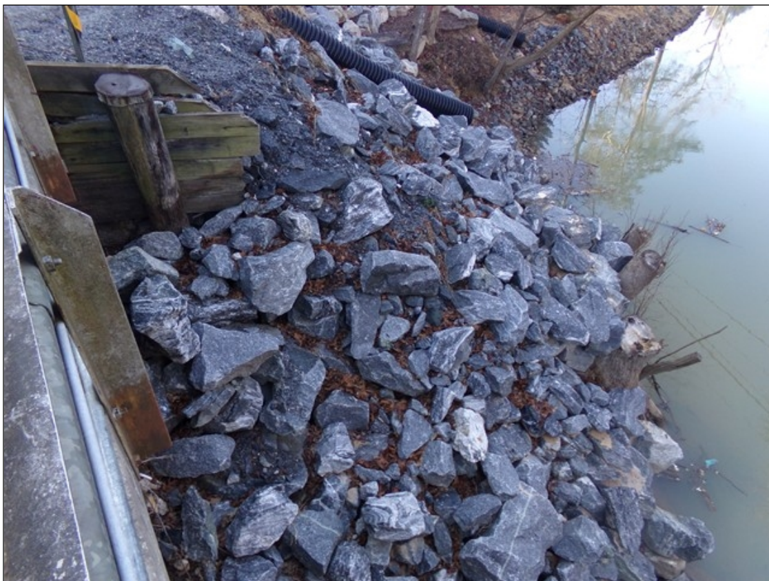
NEWLY PLACED RIP-RAP SLOPE PROTECTION AND SOUTHWEST BANK ADJACENT TO BRIDGE
