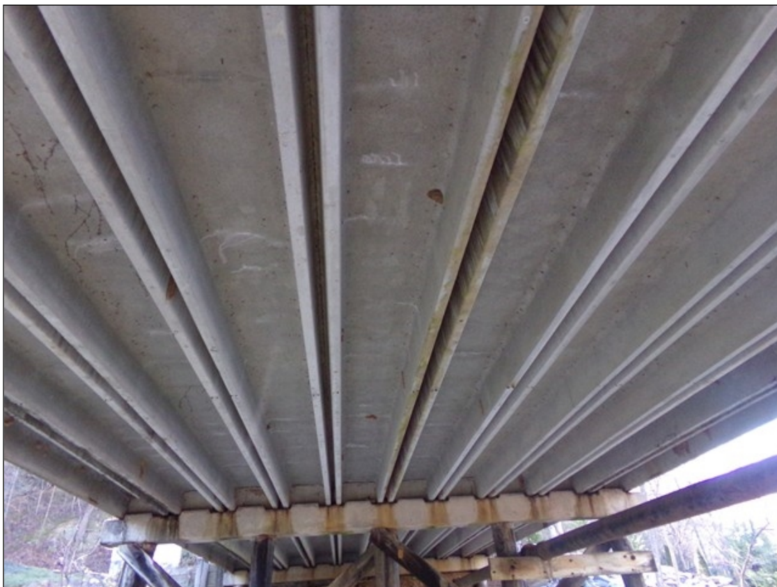
TYPICAL SUPERSTRUCTURE, SPAN 2 LOOKING BACK
