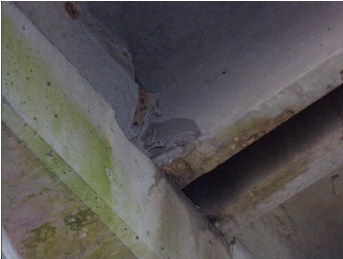
SPAN 2 BEAM 2 - SOUND PATCH (5 INCHES X 5 INCHES) TO LEFT FACE OF RIGHT LEG AT FAR END
